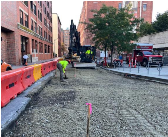
Backfilled and regraded roadway.
