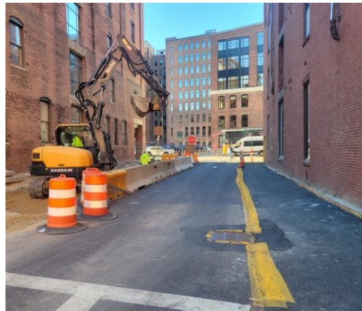
Flipped the work zone to the southeastern side of Sleeper Street.
