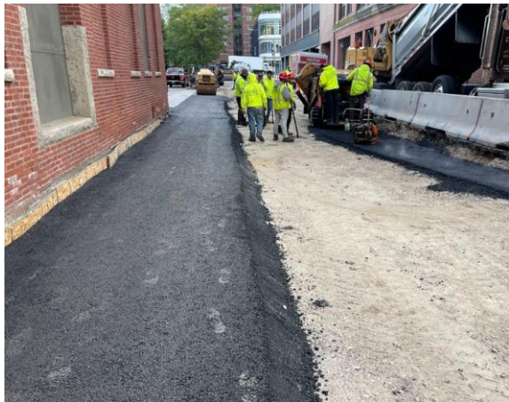
Paved roadway with binder course and installed temporary asphalt walkway.
