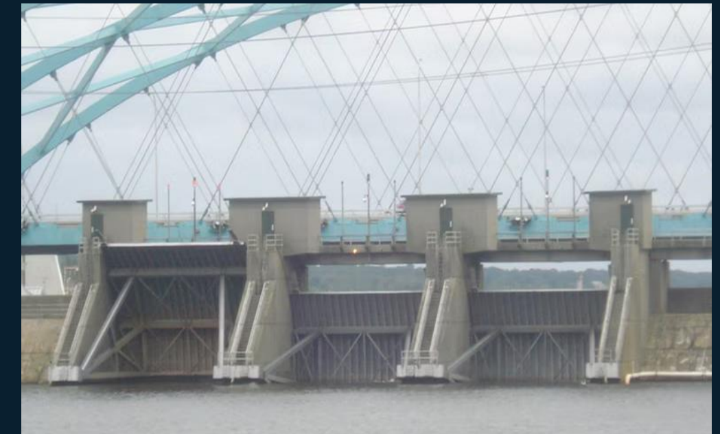
Fox Point Hurricane Barrier, Providence, RI Image source: USACE, New England District
