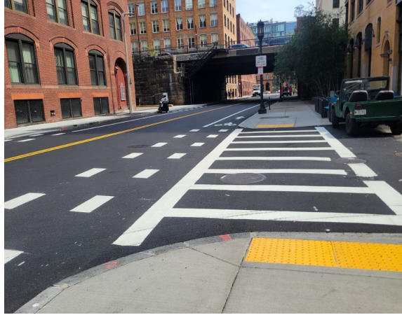
Installed striping on A Street.
