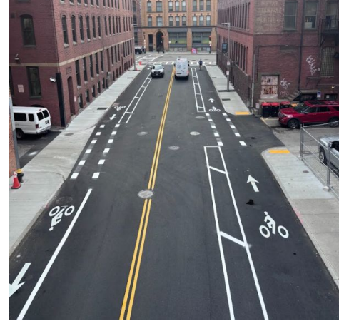
Substantially completed A Street on schedule.
