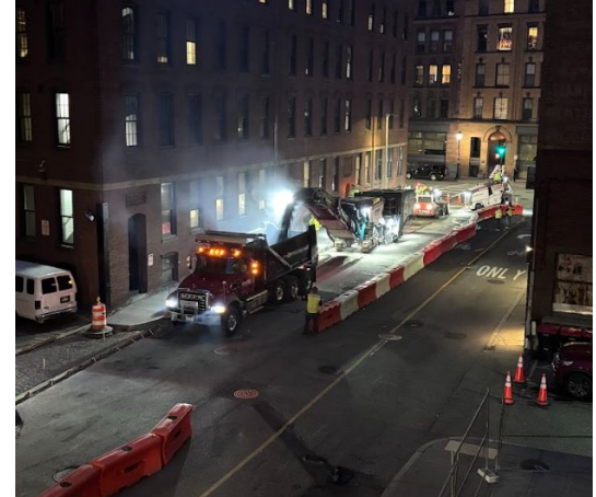
Milled the roadway on A Street and prepared for repaving.
