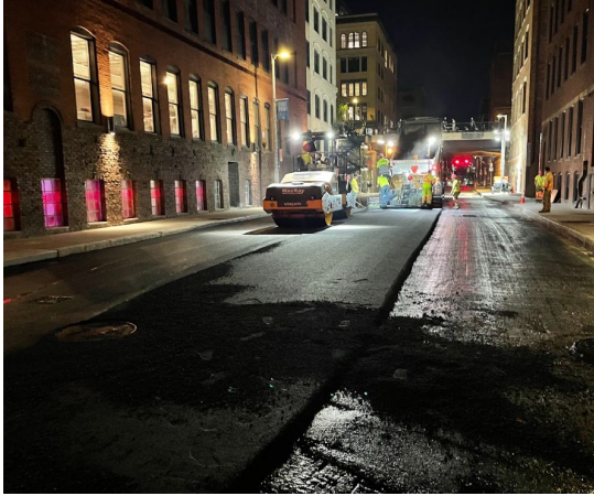
Repaved A Street.
