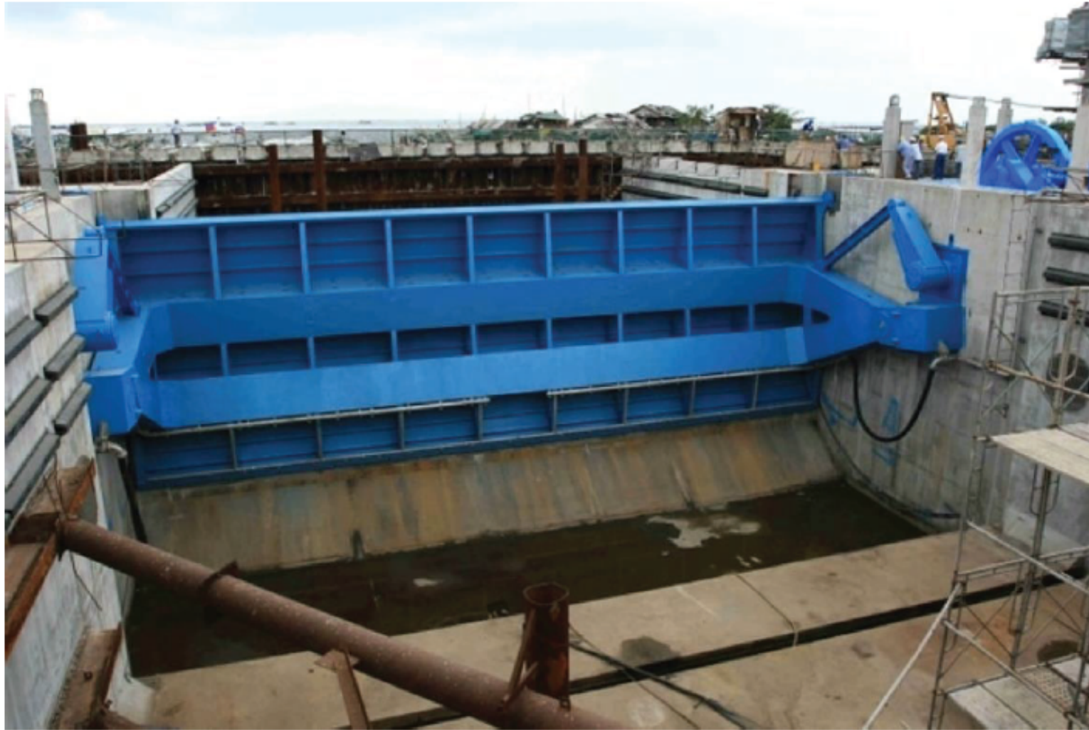
Kamanava submerged tainter gate (in dewatered condition), Kamanava, Philippines
