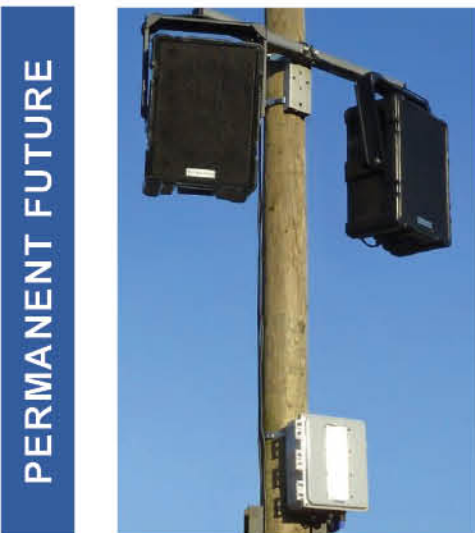
SPO1 (4) Permanently Installed Speakers & Amplifiers
