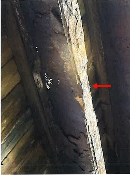
South Bay, Btw FB24 & FB25 – Stringer S2 (2024)
