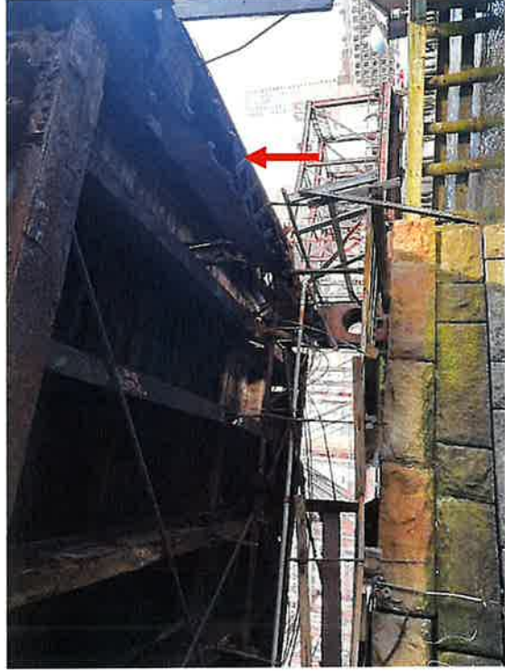
North Truss at L23L24 (2024)
