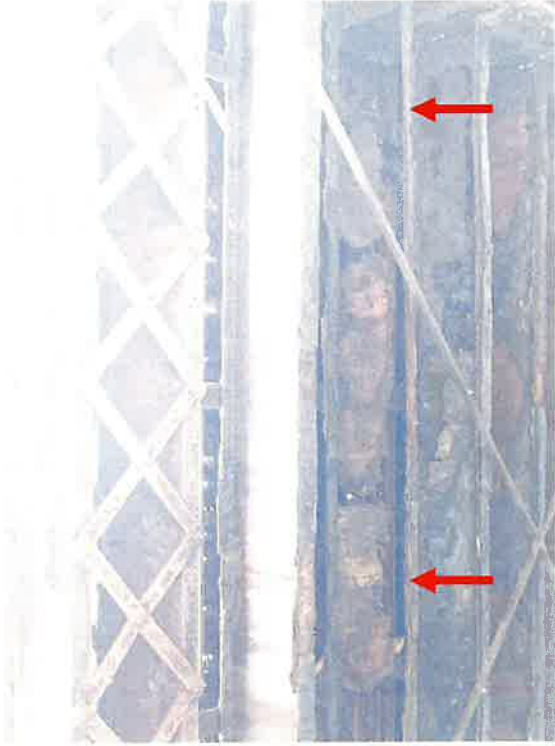
Swing Span, North Bay, Btw FB10 & FB11 – Stringer S3 (2024)
