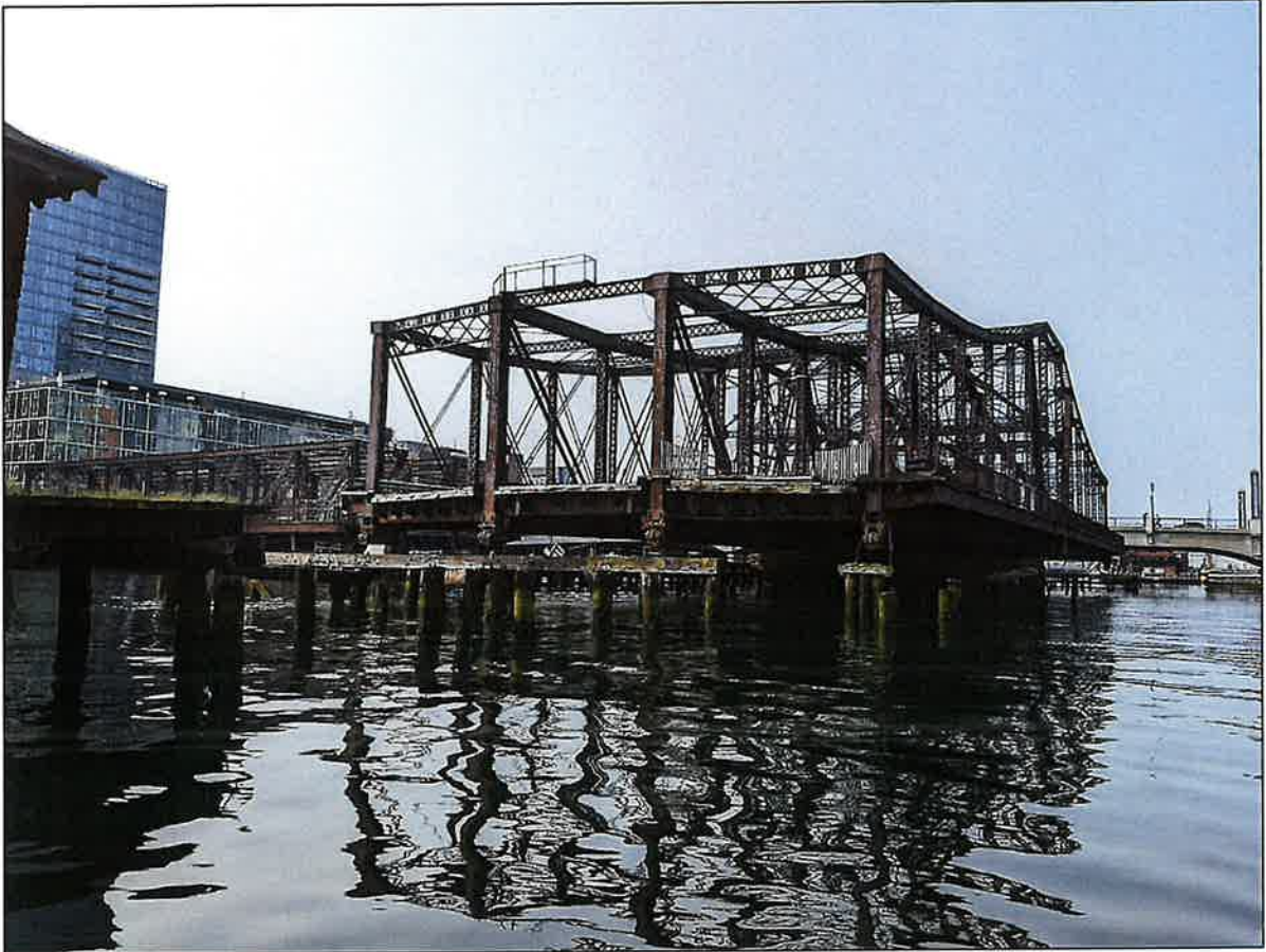
Photograph 2: North portal of open swing span, looking south. Note the unsupported ends of the swing span (August, 2024).
