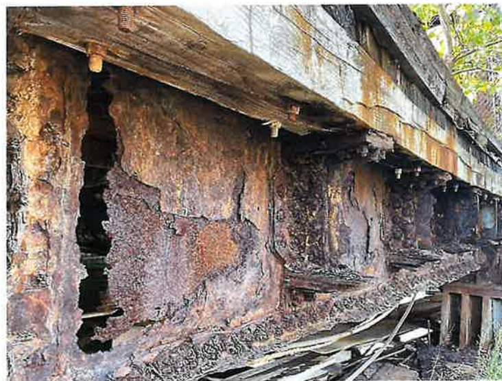
Photo 14: Approach Span 2, Pier 2, Floorbeam FB23 (Looking East)
