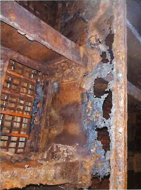
Swing Span , North Bay - Floorbeam FB17 (2017)
