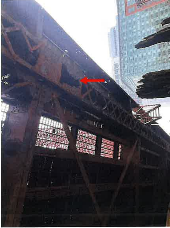
North Truss at L17L18 & L18L19 (2024)
