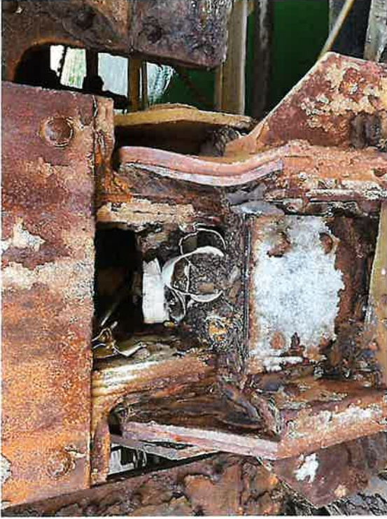
Pier 2, Center South Truss L23 Bearing (2024)
