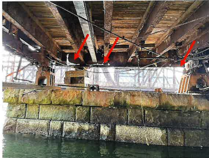
Photo 13: Approach Span 1, Pier 1, Floorbeam FB8 (Looking East)
