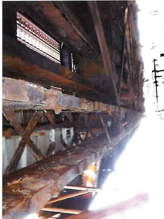
North Truss at L16L17
