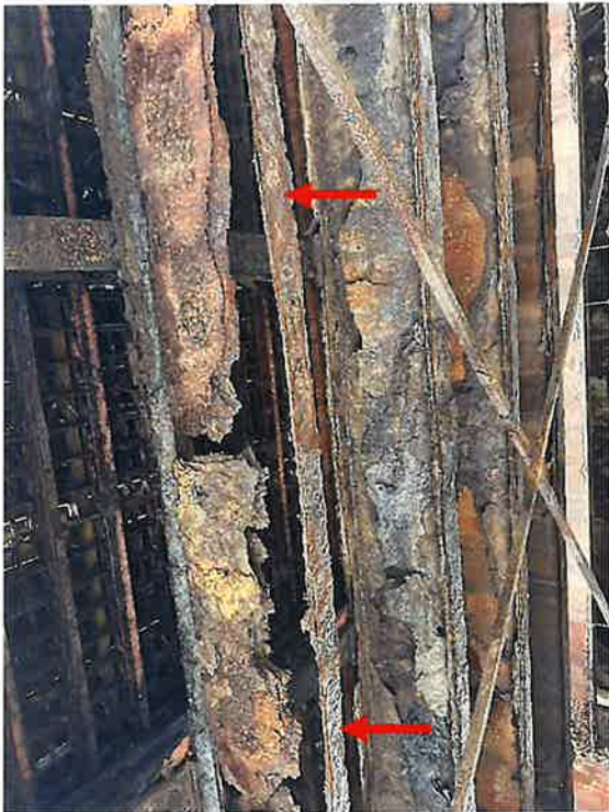
Swing Span, North Bay, Btw FB10 & FB11 – Stringer S2 (2022)
