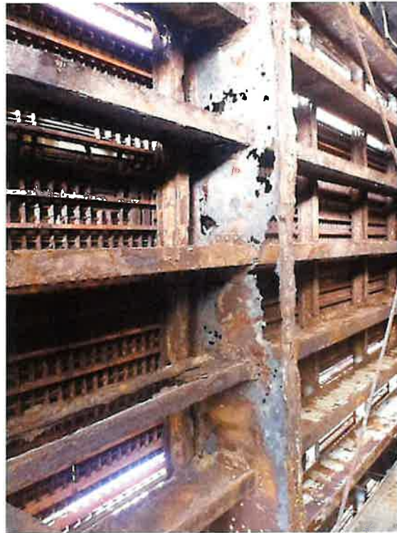
Swing Span, North Bay - Floorbeam FB10 (2017)
