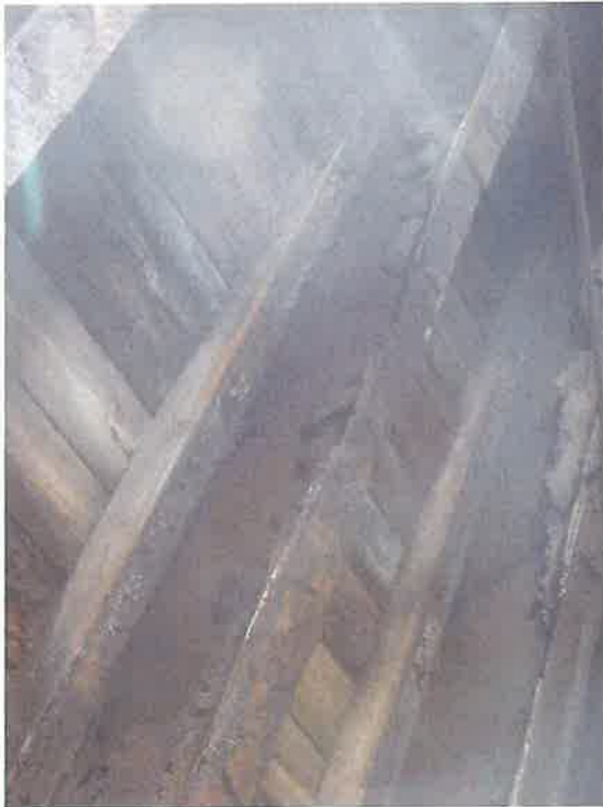
South Bay, Btw FB24 & FB25 – Stringer S2 (2017)
