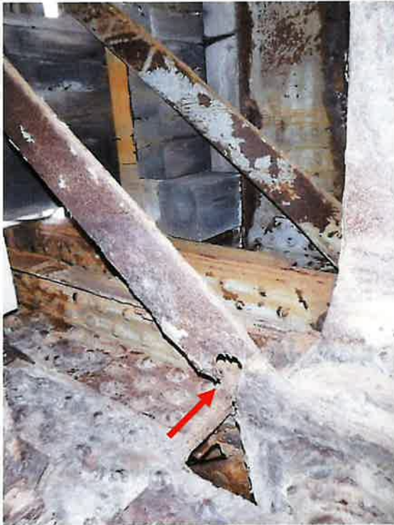
Center North Truss at L26U27 at L26 (2017)
