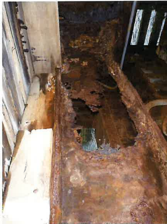
South Bay, Btw FB23 & FB24 – Stringer S1 (2017)
