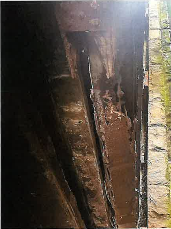
Center South Truss at L1-L2 (2022)
