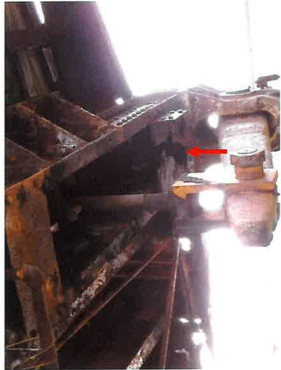
North Truss at L9L10 at L9 (2017)
