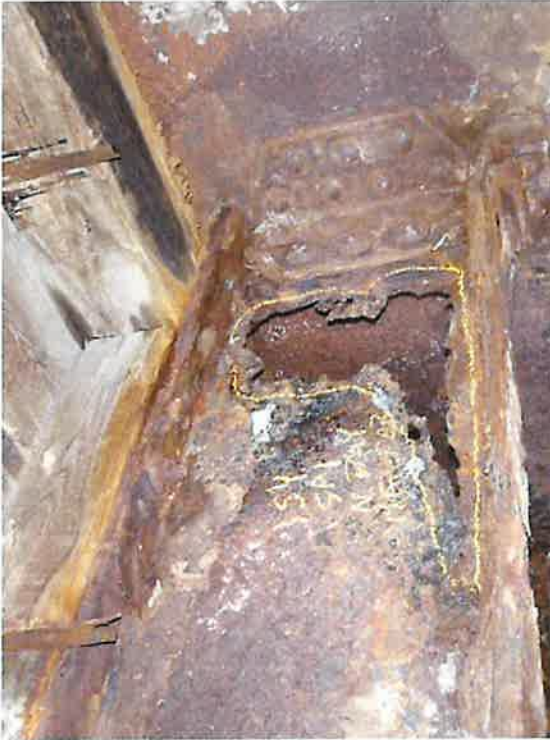
North Bay, Btw FB2 & FB3 – Stringer S4 (2017)
