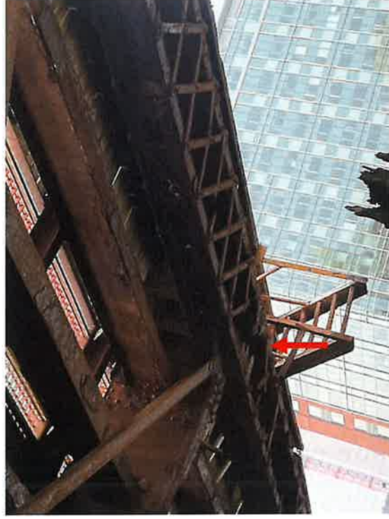
North Truss at L16L17 (2024)
