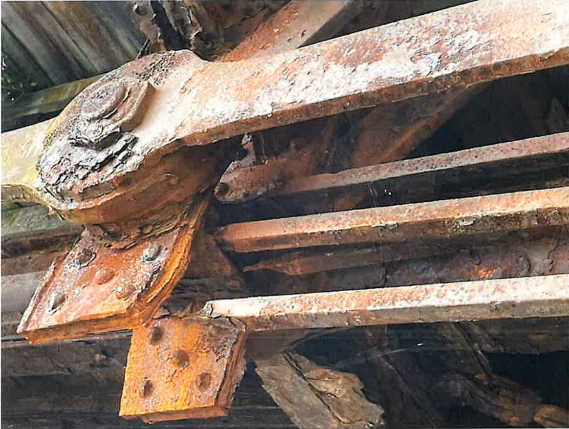
Photo 2. Span 1, North Truss, Lower Chord, L2-L3 (Looking East)
