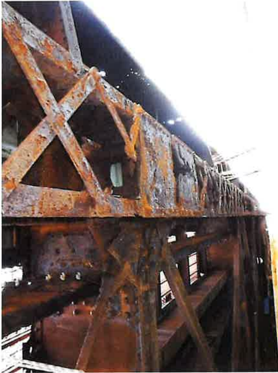
North Truss at L17L18 & L18L19 (2017)
