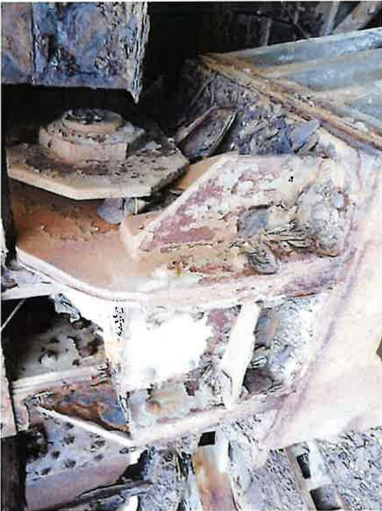
Pier 2, Center South Truss L23 Bearing (2017)
