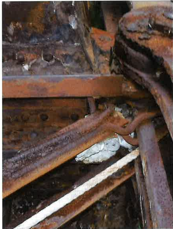
North Truss- L4U5 at L4 (2017)
