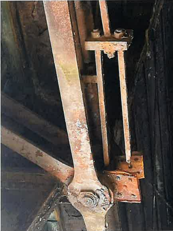
North Truss at L2-L3 (2022)
