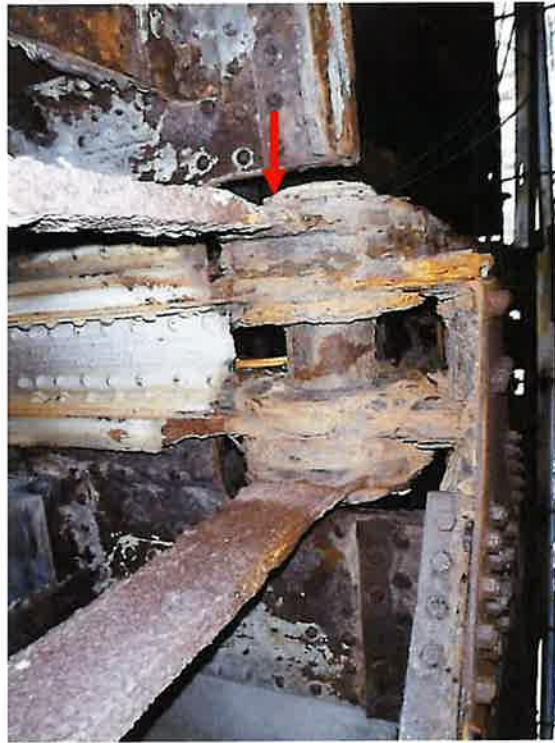
Center North Truss L24L25 at L24 (2017)
