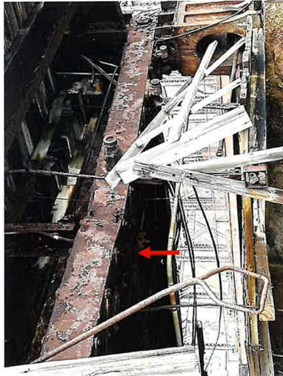
North Truss at L23L24 (2022)
