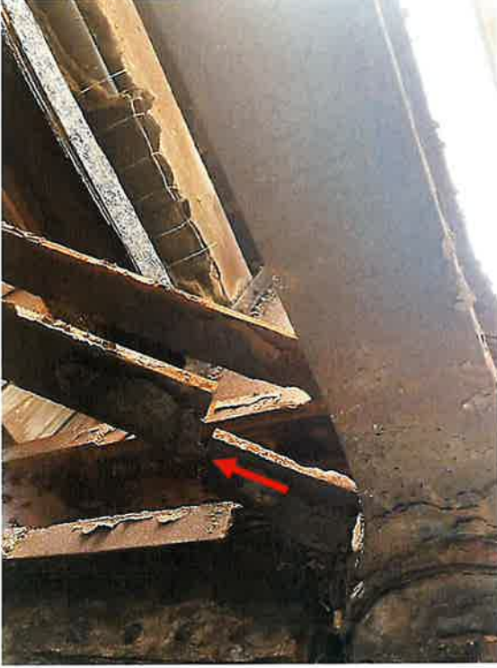
North Truss at L27U28 at L27 (2024)
