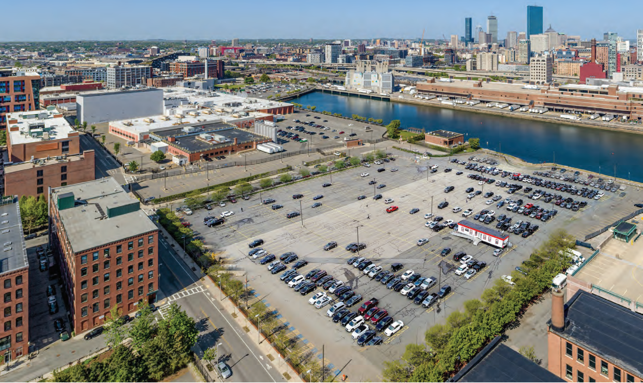
6.35 Acres of Flood-prone Impervious Parking Lot with over 800 Cars
