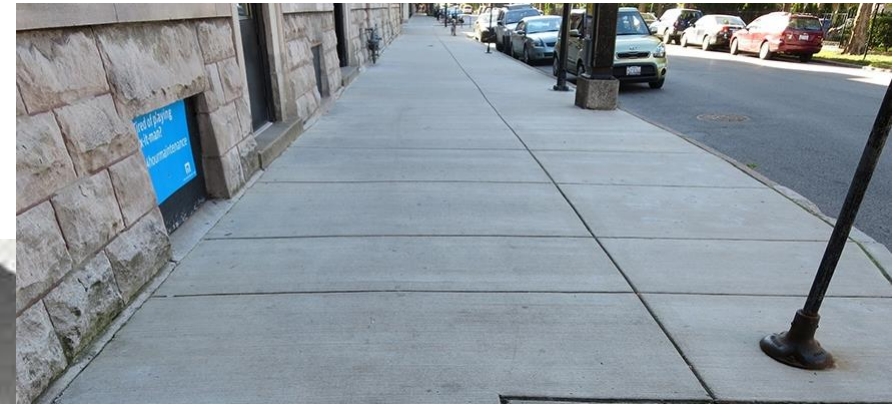
Example concrete sidewalk and vertical granite curb
