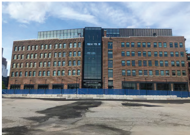
View of 5 Necco Street building from the Project Site looking north
