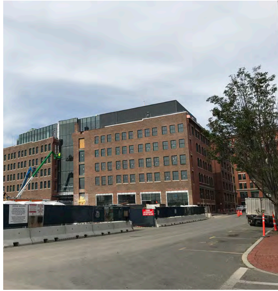
View of 5 Necco Street building from Necco Street
