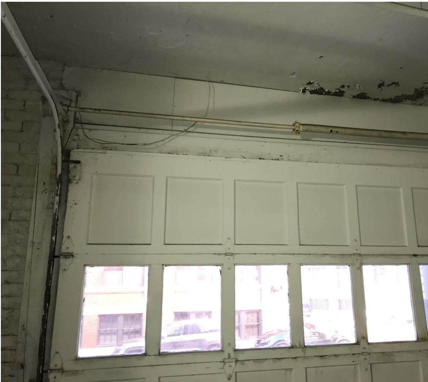
**OPENING #5 EXISTING INTERIOR JAMB, HEADER AND TRACK DETAIL**
