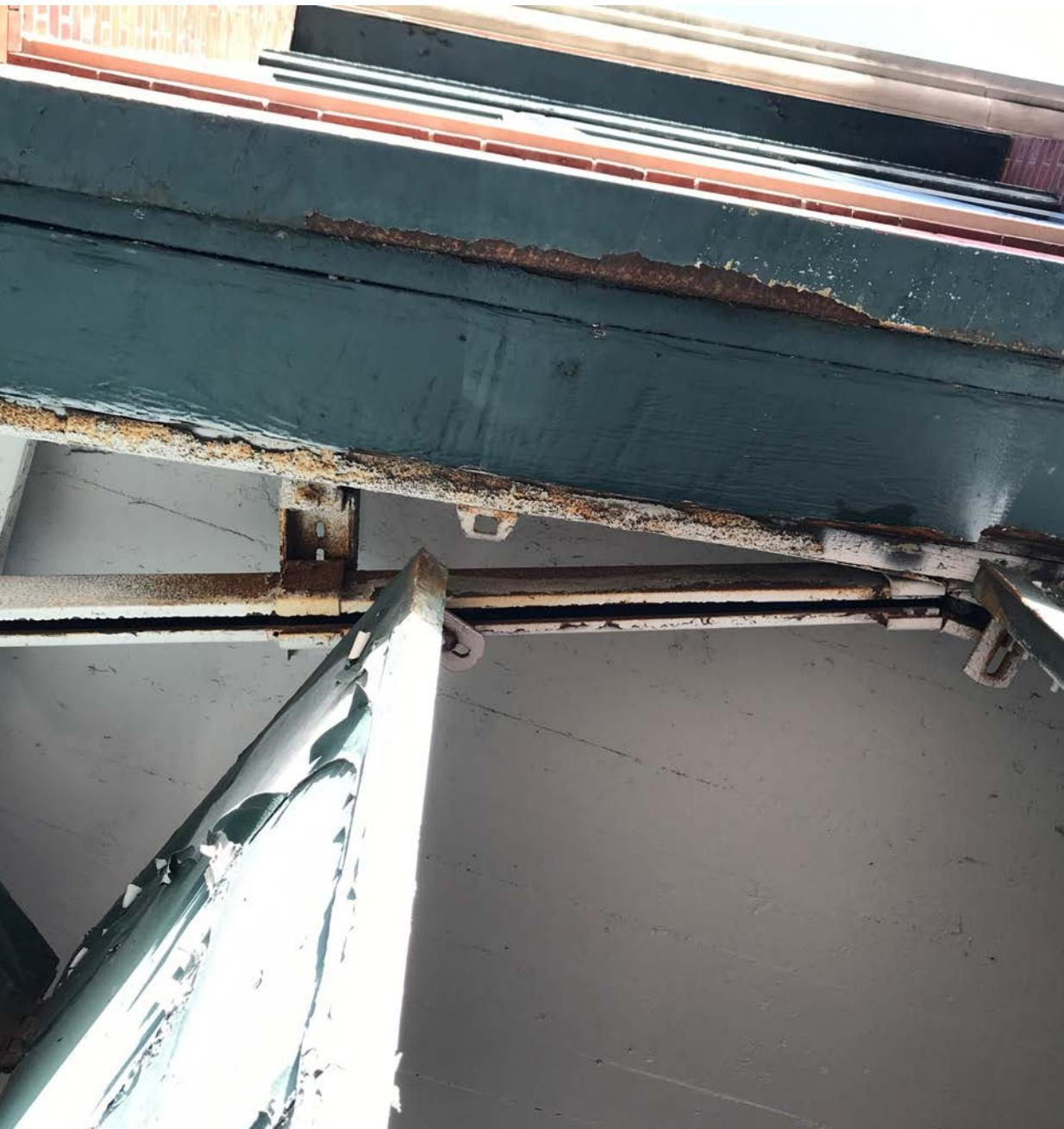
OPENING #2 EXISTING EXTERIOR HEADER & INTERIOR TRACK DETAIL
