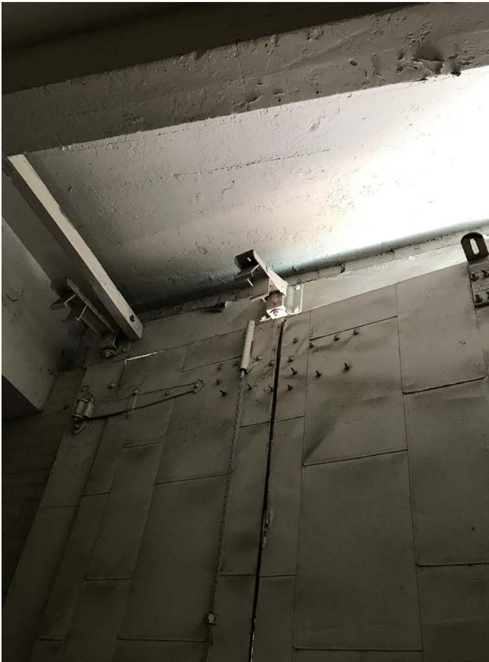
OPENING #3 EXISTING INTERIOR TRACK AND HEADER DETAIL
